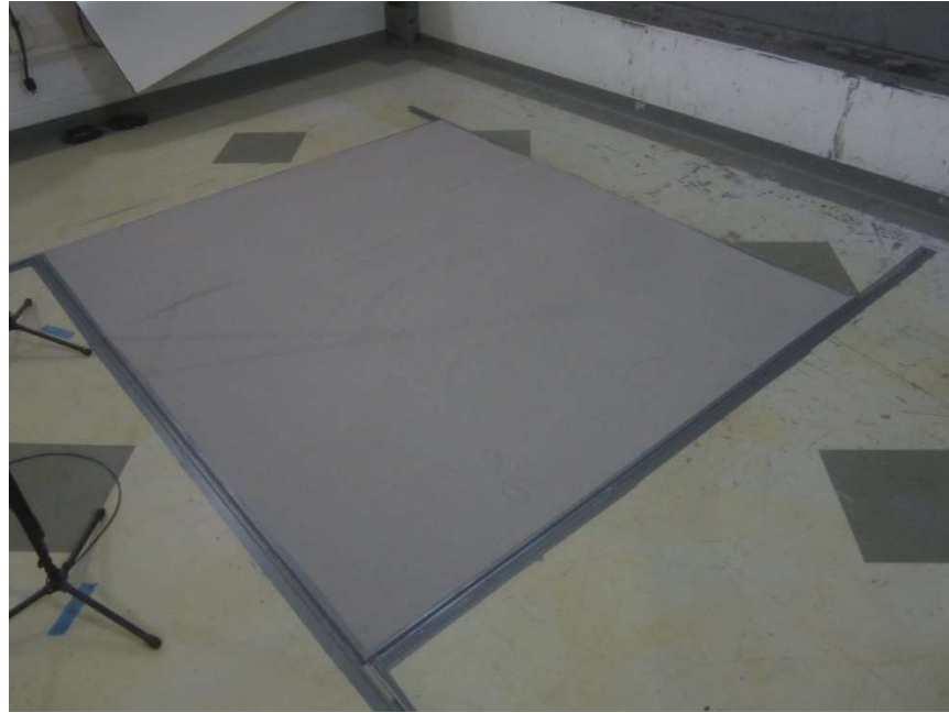
Installed Specimen Midway Mineral
